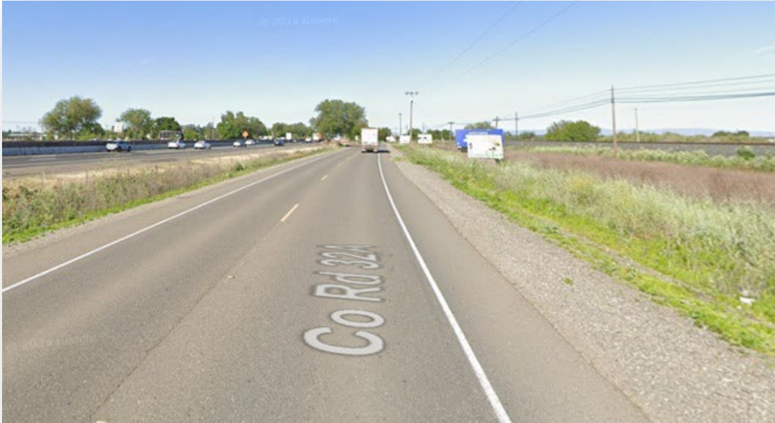
Figure 15: County Road 32A Existing Conditions
