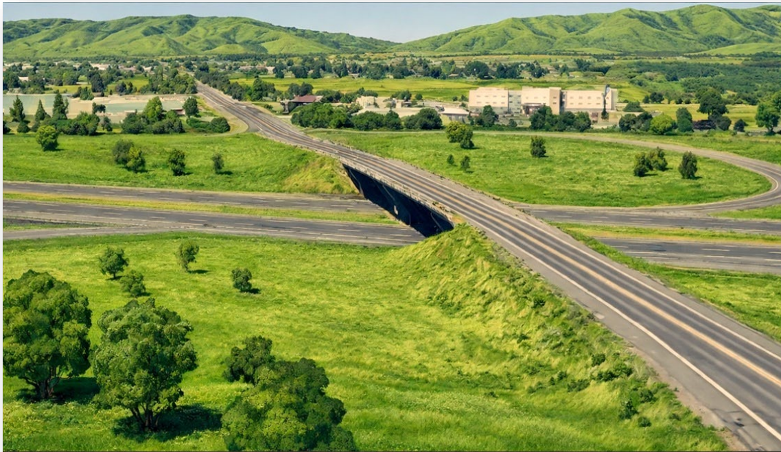
Figure 9: Grant Ave / I-505 Overcrossing Existing Conditions
