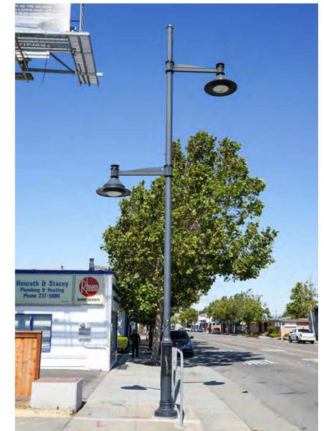
Figure 42: Street lighting featuring dedicated illumination for both the roadway and the sidewalk
