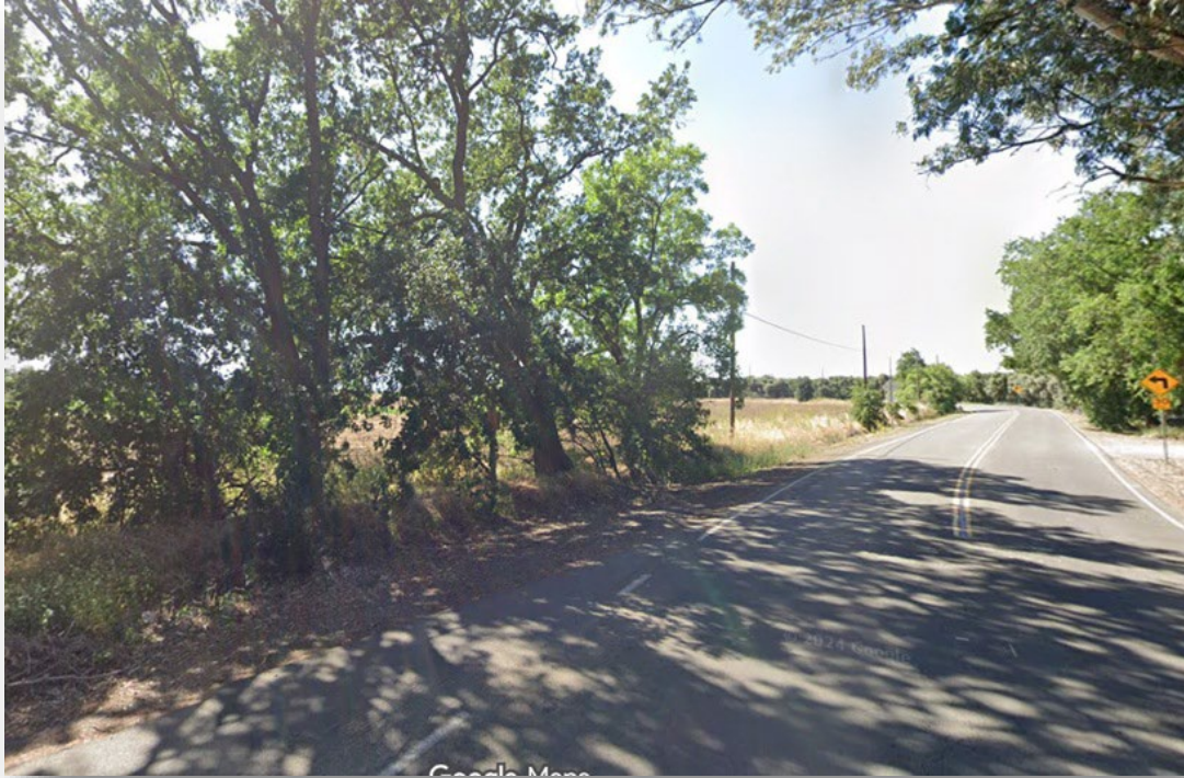
Figure 108: Russell Blvd @ Stevenson Bridge Road Existing Conditions
