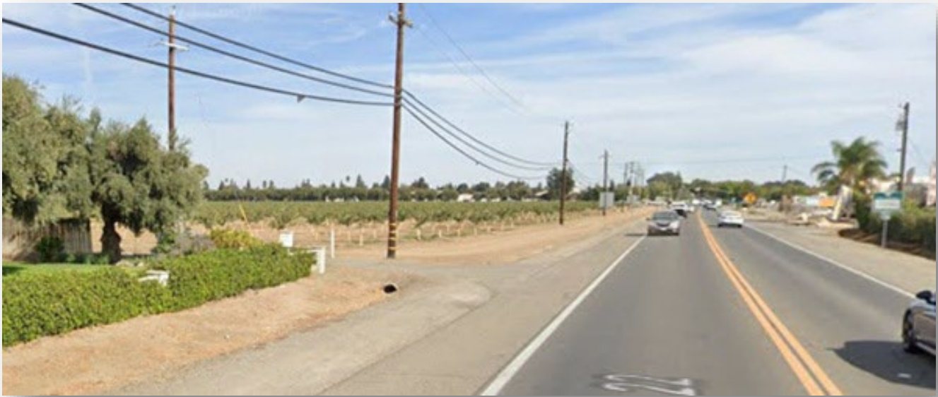
Figure 21: SR-16 Eastbound Approaching County Road 98 Existing Conditions
