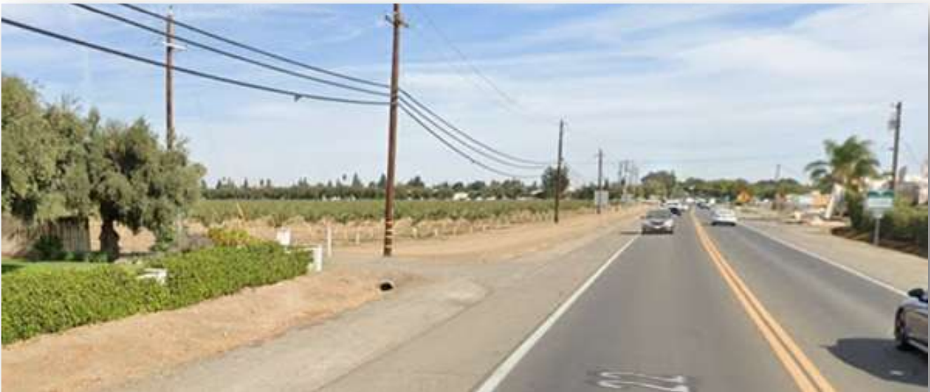
Figure 21: SR-16 Eastbound Approaching County Road 98 Existing Conditions
