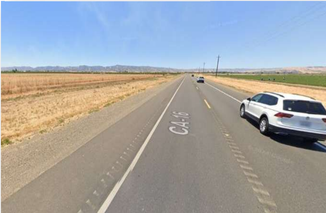
Figure 2: CA-16 Westbound Existing Condition
